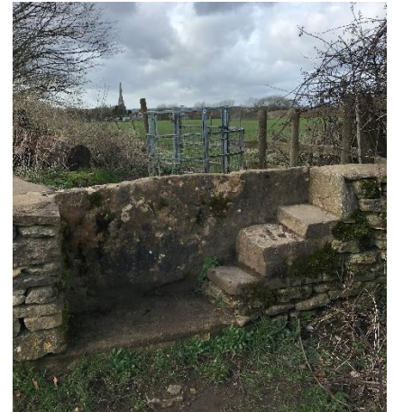
Modified and maintained
