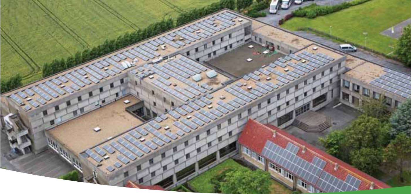
Solar panels on roof of office buildings
