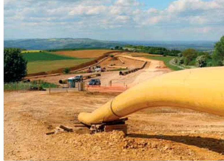
Saltway Hill during pipeline installation
